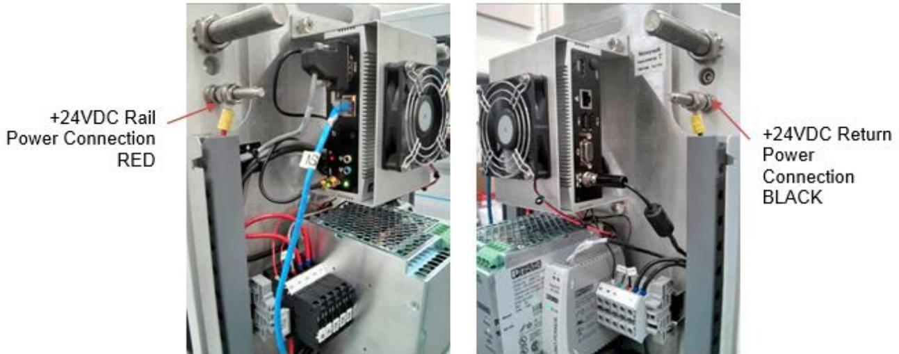
**Figure 6-9: Rail Wiring Connections**
