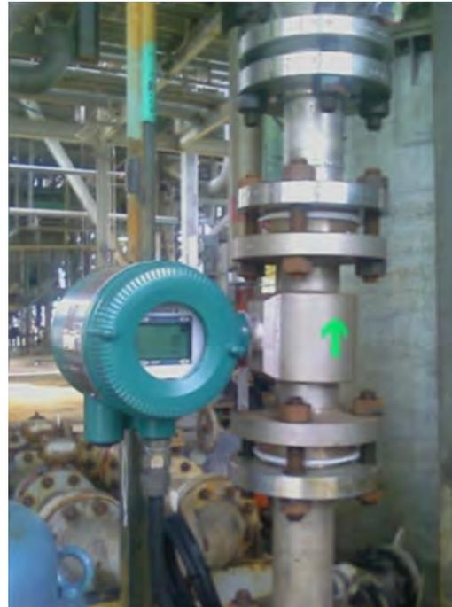
Traditional technology is not as accurate as new technology and requires more maintenance due to wear and tear on moving parts. With its two-wire technology, the ADMAG AXR magmeter presents an ideal replacement solution with no pressure loss. And with its short face to face length, pipe modifications can be kept to a minimum.
